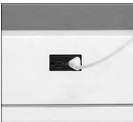
Duplex receptacles snap into raceway.
